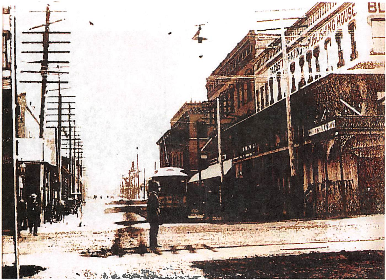
The corner of Bay and Main streets sometime after 1895 — Jacksonville now had what the people wanted. Note the arc light hung overhead, the electrified trolley car — no longer powered by horses or mules — and the lines of poles draped with dozens of electric, phone and telegraph wires.
