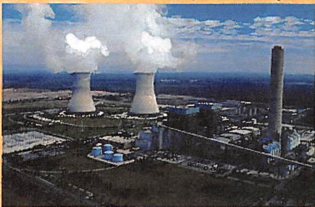
SJRPP was four months ahead of schedule and $200 million under budget — Ground was broken for the St. Johns River Power Park in 1982. As many as 2,200 workers were involved in its construction. The first unit at SJRPP was declared ready for commercial operation on March 27, 1987; the second ready on May 27, 1988. By burning coal instead of oil, SJRPP is a major money-saver for the JEA's customers.
